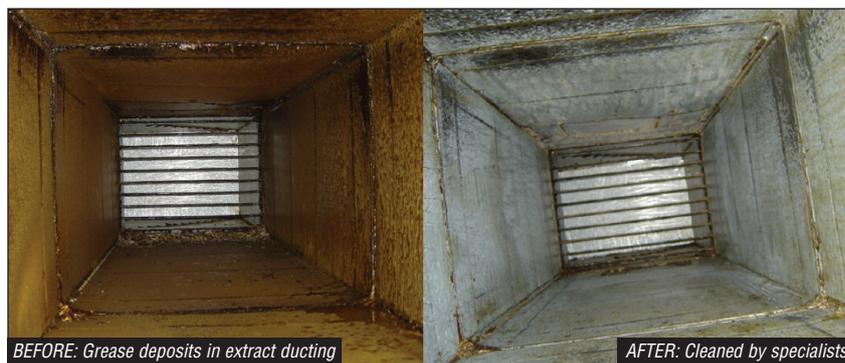
**“Grease-laden fumes from the cooking operation accumulate on the internal surfaces of the ducting requiring only a spark or flame from cookers or fryers to set fire to the grease deposits”**
