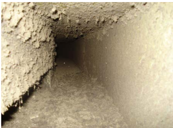
Internal duct surfaces showing accumulation of dust and debris
