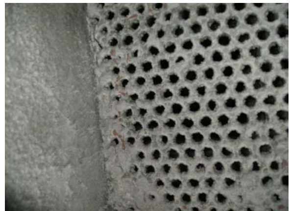
Internal duct surfaces showing accumulation of dust and debris
