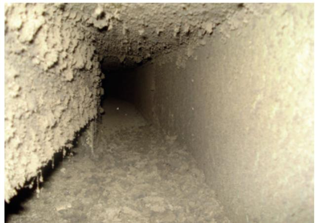
Internal surfaces of air conditioning duct showing accumulation of dust and debris
